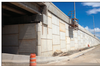
Access Ramps for Mall of San Juan San Juan, Puerto Rico
