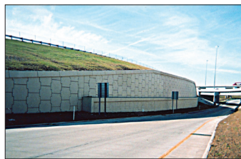
I-70 / I-270 MSE Wall Support Hazlewood, Missouri, USA
